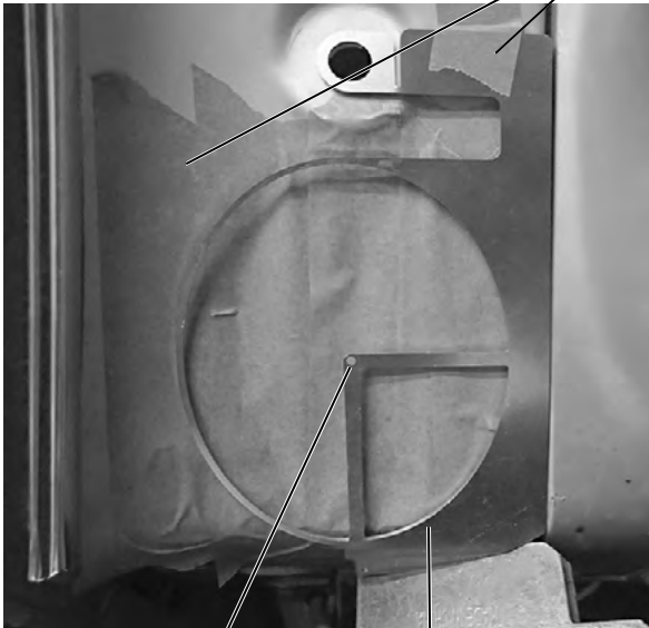
Use Center Punch to Mark Dash (For Standard Louvers)
